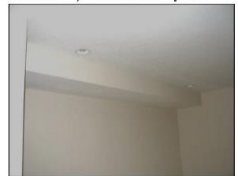
Figure 3. New Tradition Homes – Ducts Between Floors, Pre- and Post-Drywall
