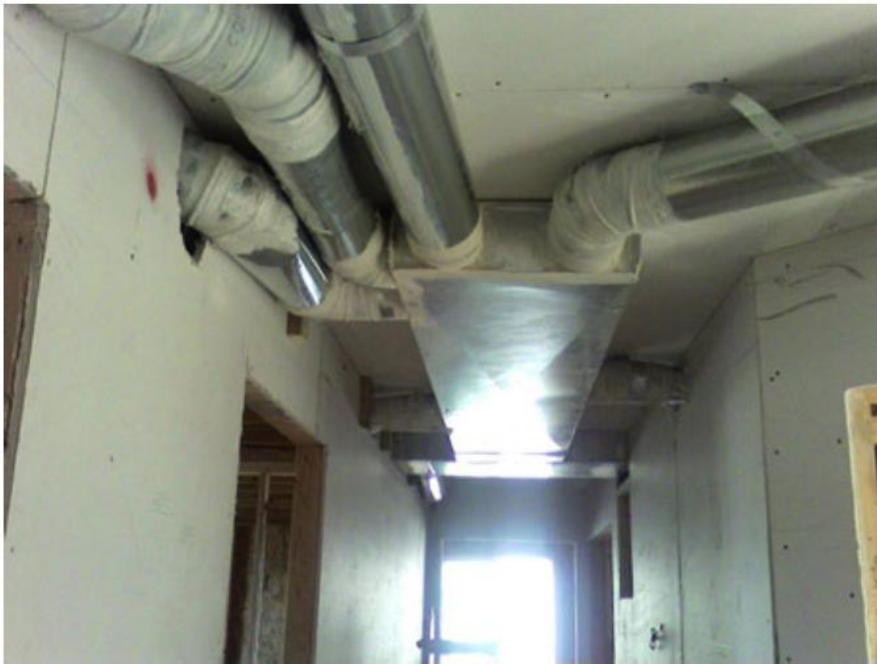
Figure 1. Habitat for Humanity, Moses Lake - Duct Chase Pre- and Post-Drywall
