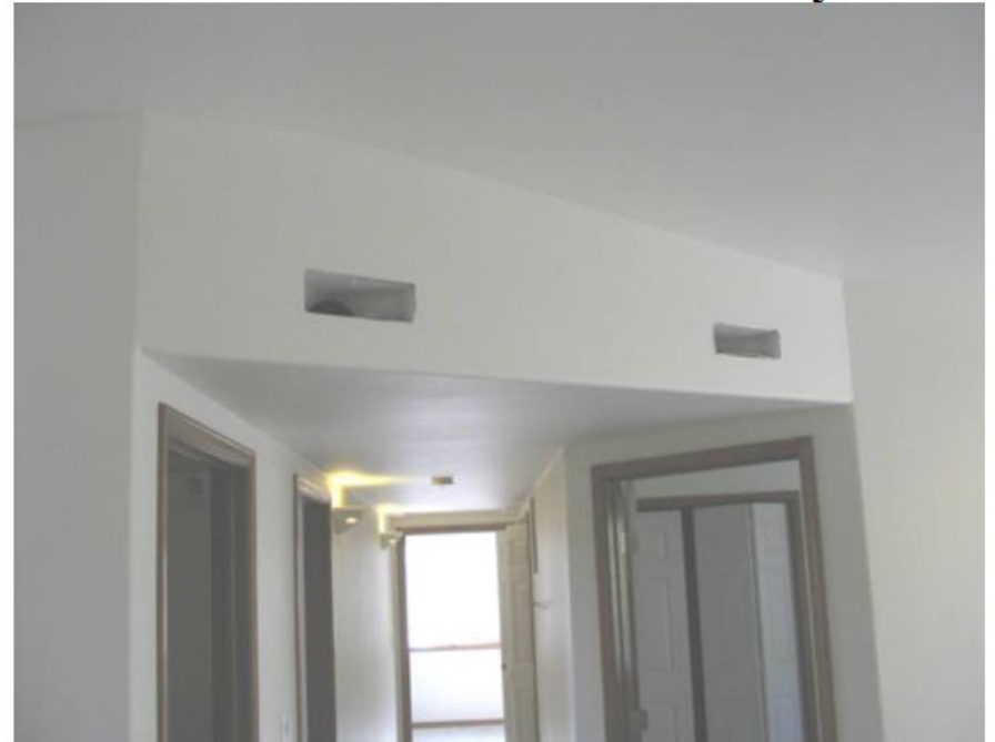
Figure 1. Habitat for Humanity, Moses Lake - Duct Chase Pre- and Post-Drywall
