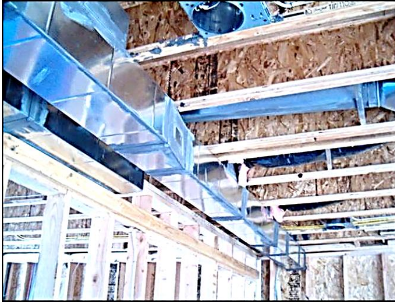
Figure 5. New Tradition Homes – Air Handler in Conditioned Space, under Stairwell
