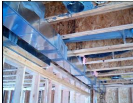
Figure 3. New Tradition Homes – Ducts Between Floors, Pre- and Post-Drywall
